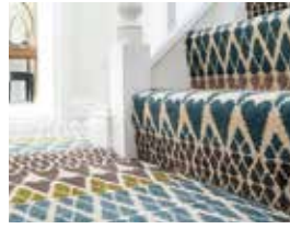
Private Villa, Abu Dhabi Installing carpet flooring
